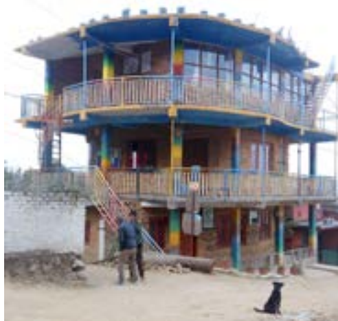
Nepal: the KRMEF's school building
